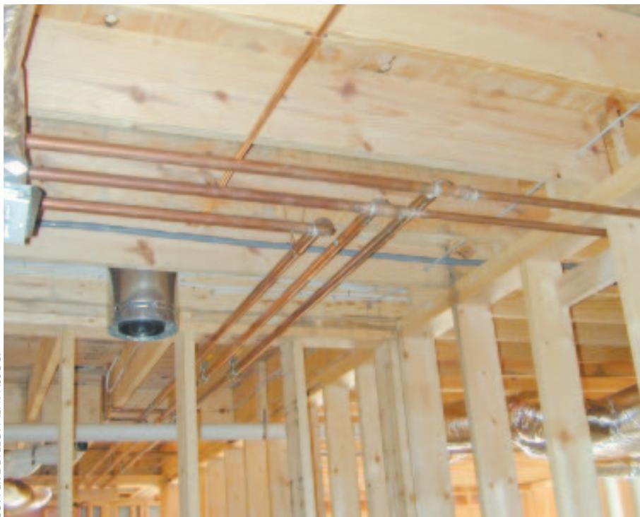
**Figure 5.** In this home,  $3/4$ -inch copper lines tee off from the 1-inch mains on the left.
